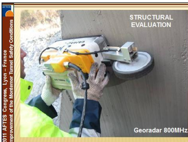
Figure 8: Structural evaluation using georadar
