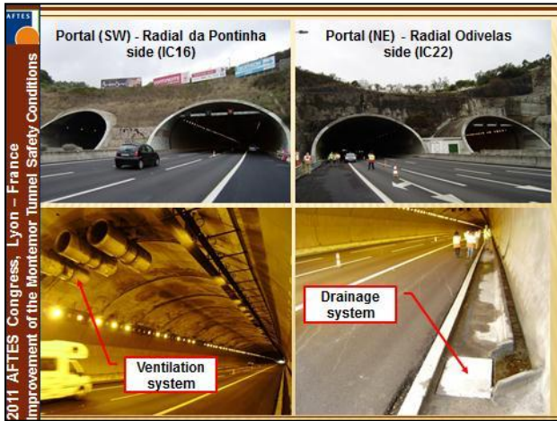
Figure 2: View of the tunnel portals, as well as of both the existent ventilation and drainage systems
