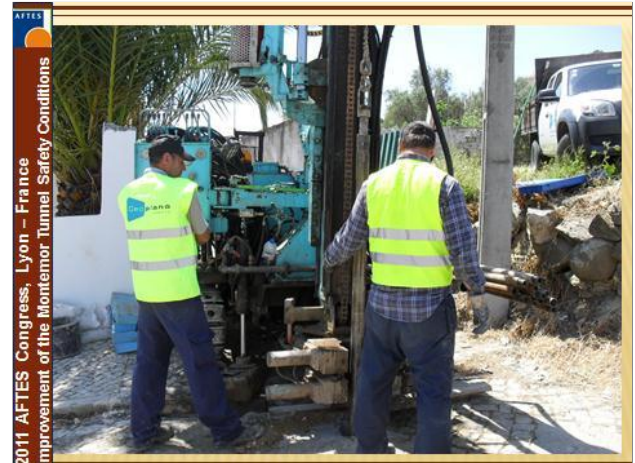
Figure 9: Piezometer installation
