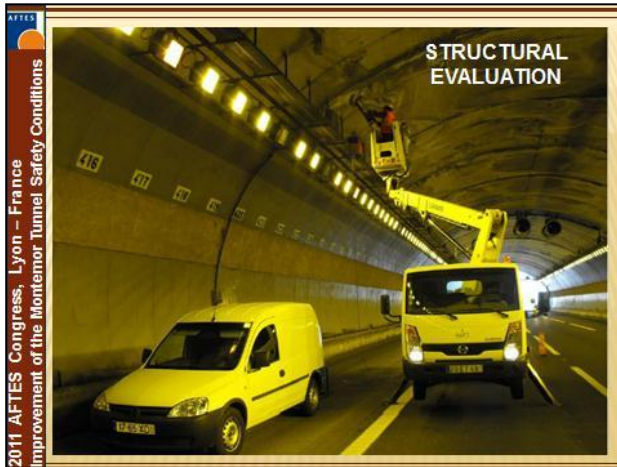
Figure 7: Tunnel structural evaluation
