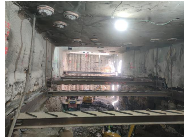
Jet grouting columns
