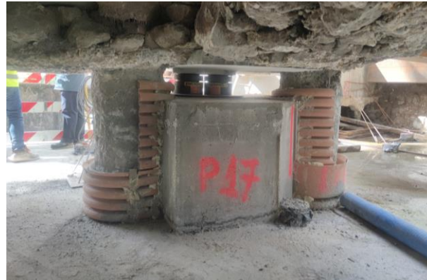
Sheathing of the piles
