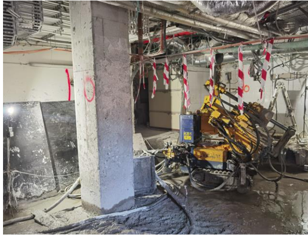
Execution of jet-grouting columns
