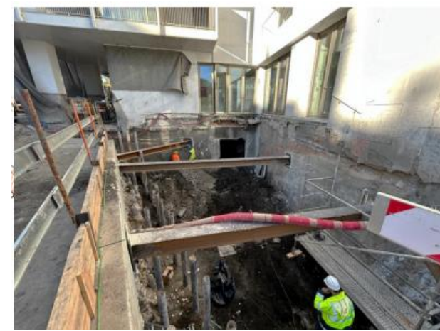
Installation of steel struts first level
