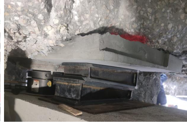
Fitting temporary wedges
