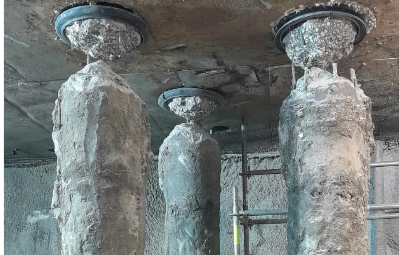
Existing bored piles demolition
