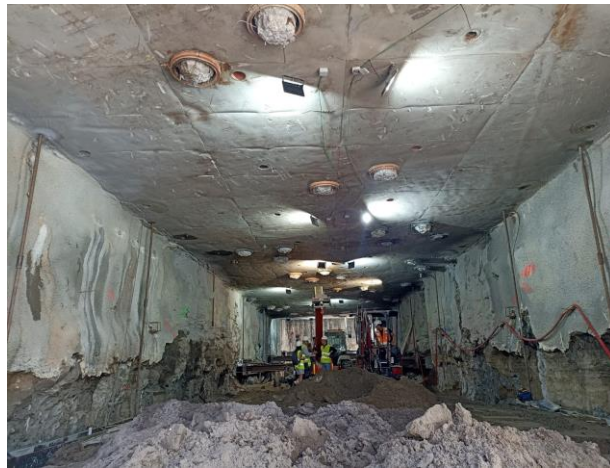
Excavation under the underpin slab level
