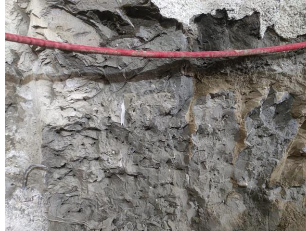
Jet grouting columns
