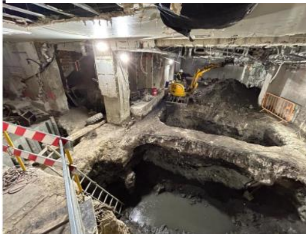
Execution of jet-grouting columns
