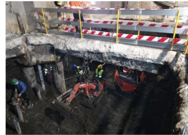
Installation of steel struts first level
