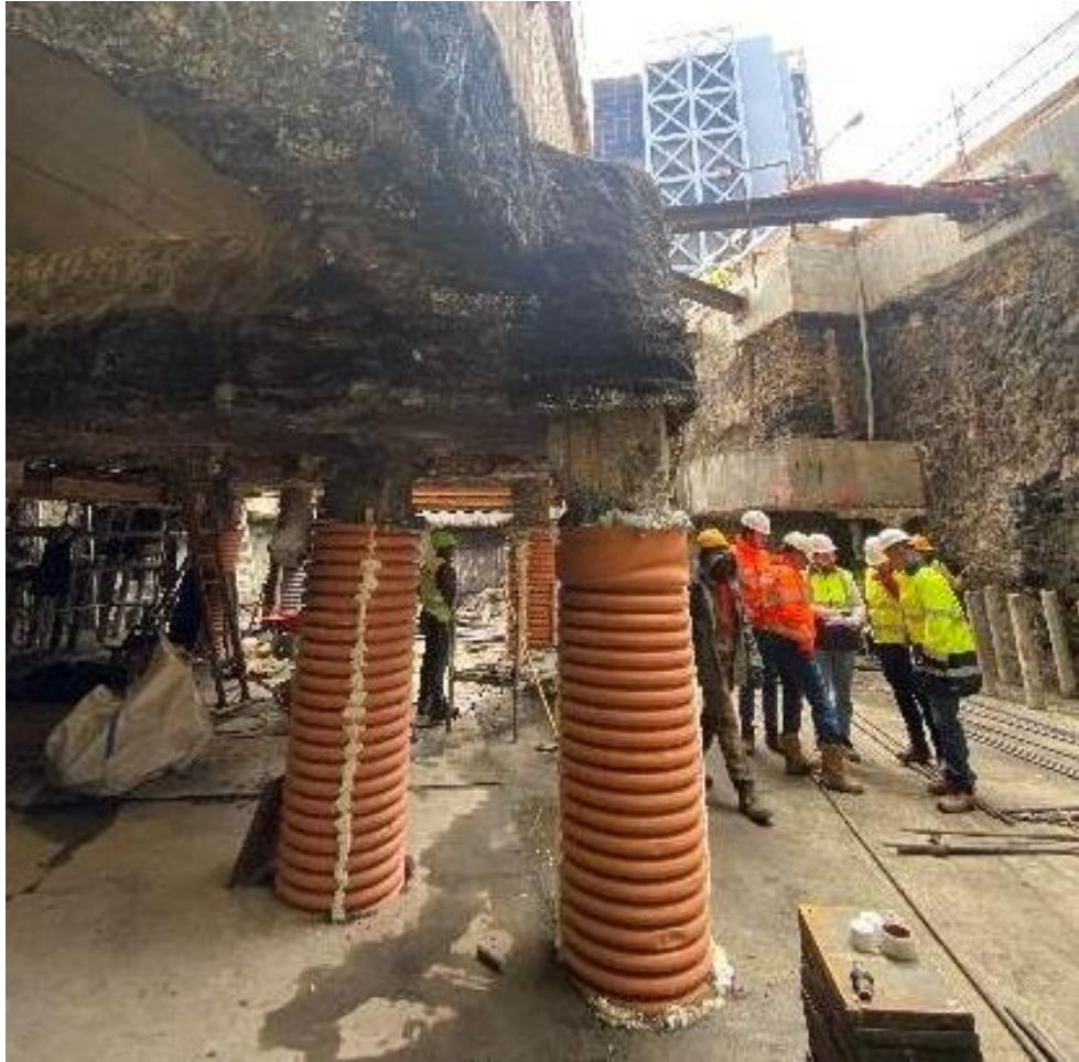
Existing bored piles casing at underpin slab level
