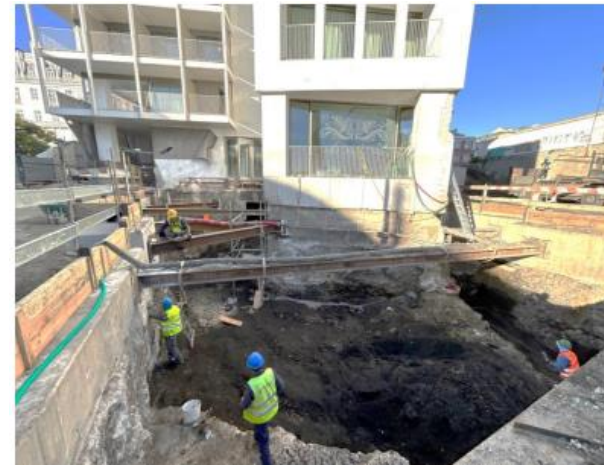
Installation of steel struts first level
