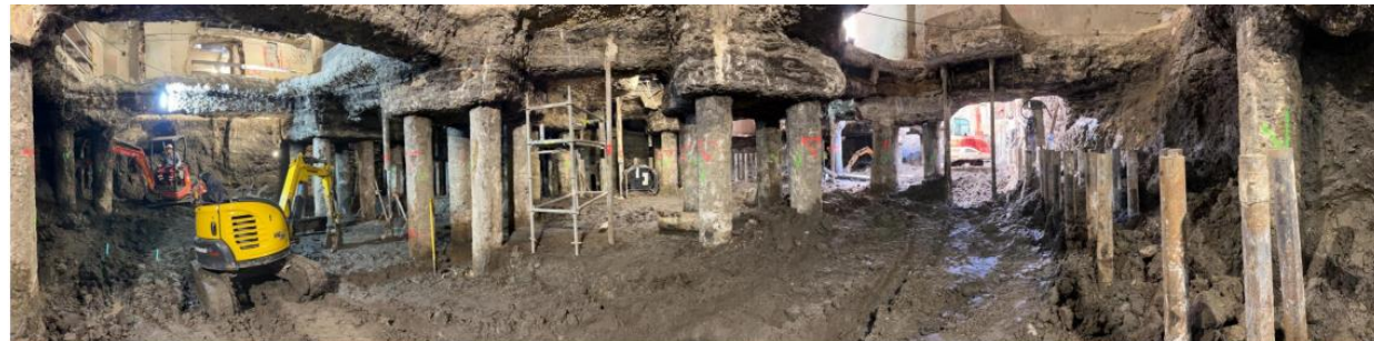
Excavation work at the existing foundation piles area
