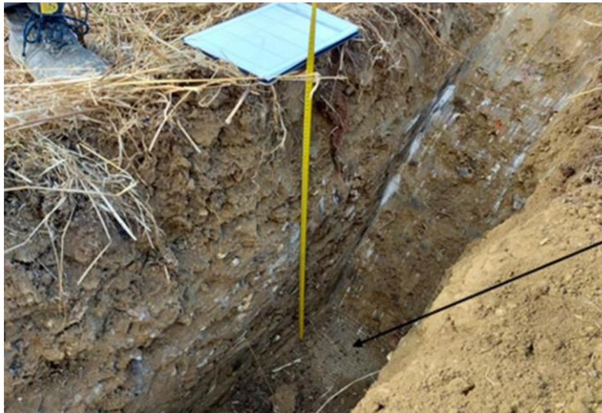
Geomembrane covering the waste landfill materials
